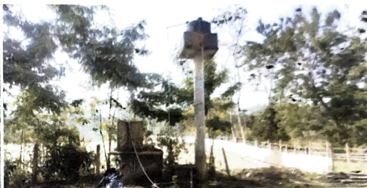
Over head tank
