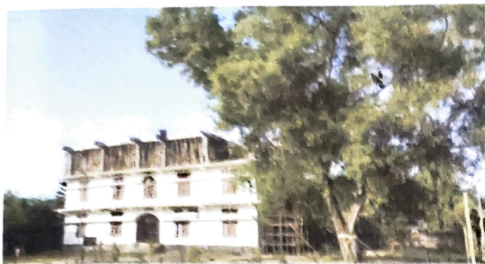
A building of the college under construction
